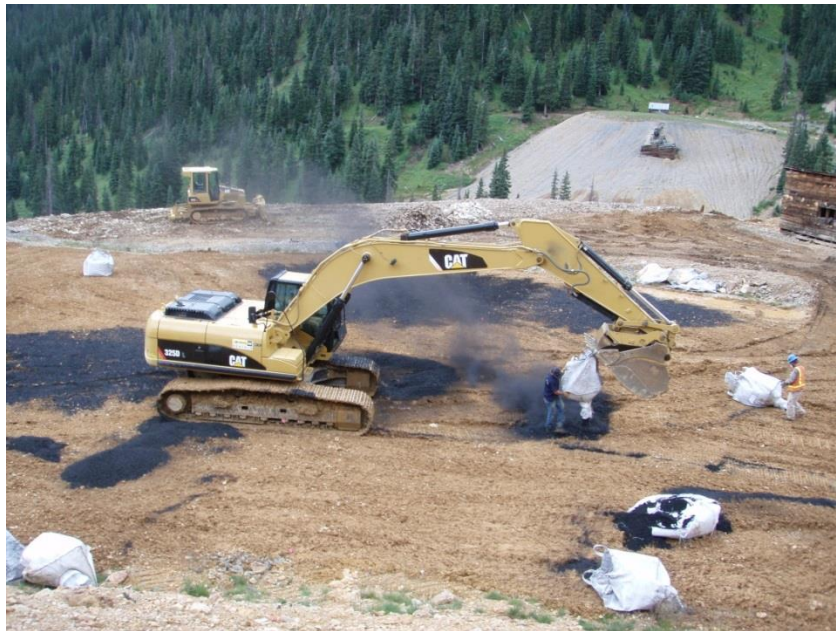
Figure 43. Biochar application at the Joe John site.
