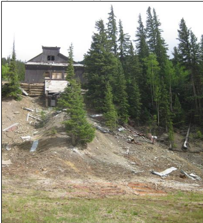
Figure 17. Lackawanna mill site
