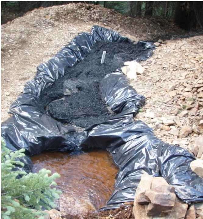
Figure 14. Biochar flume at Bonner draining adit.
